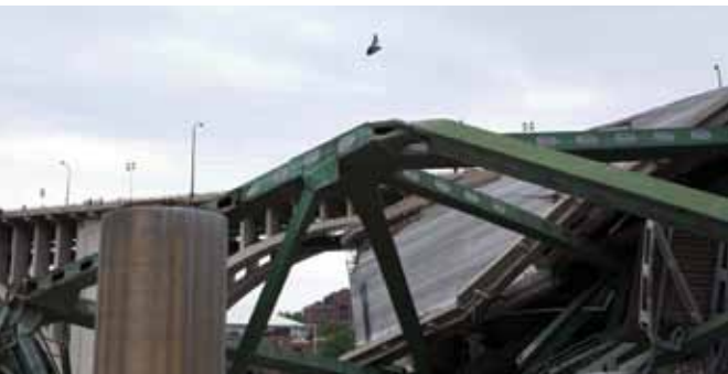
THE COLLAPSE OF THE I-35W BRIDGE IN MINNEAPOLIS TOOK THE LIVES OF 13 PEOPLE.
